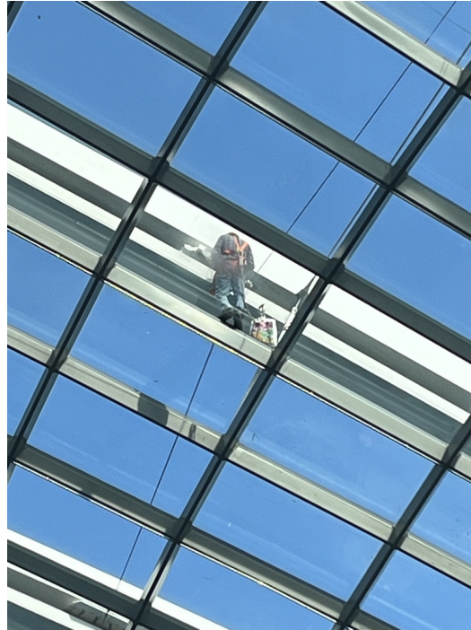
Figure 20: A worker on the dome of Flower Dome. Photo: Nadine Chan.
