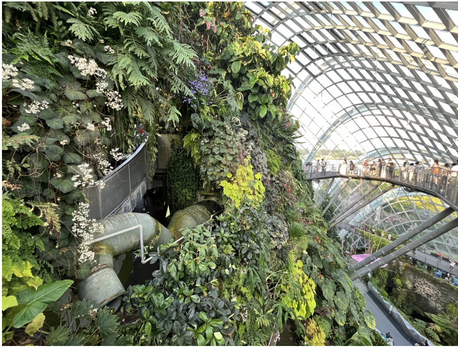
Figure 14: Mimicking the termite mound, air shafts obscured among the foliage on the mountain side of Cloud Forest help displace and diffuse air. Like the stinkhorn mushroom, the interior of the “mountain” structure is hollow, mostly supported by its latticelike outer “shell.” Photo: Nadine Chan.
