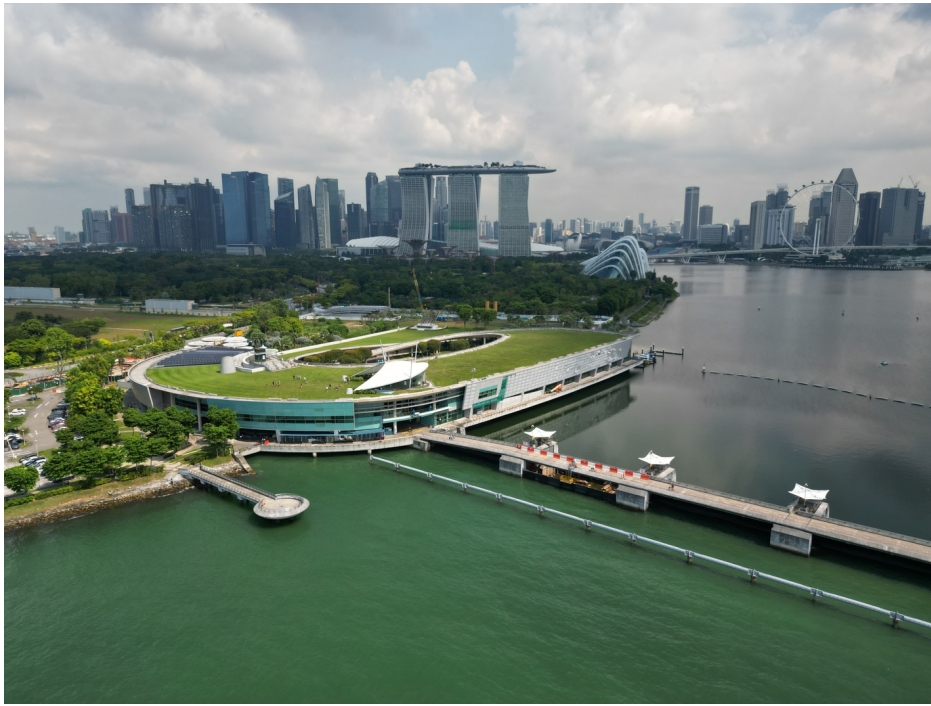
Figure 5: The Marina Barrage in the foreground transforms the tidal estuary into a freshwater reservoir that feeds the Gardens and biomes (visible in center background). The financial district is in the far background. Source: Bob Tan, CC BY-SA 4.0, https://creativecommons.org/licenses/by-sa/4.0 , via Wikimedia Commons.
