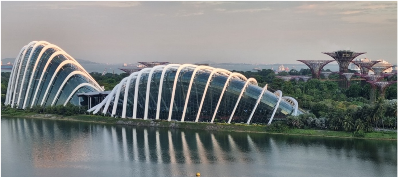
Figure 1: Exterior view of Cloud Forest ( left ) and Flower Dome ( right ). The external structural ribs add to the iconicity of the building. “Supertrees”—some of which function as chimneys releasing waste heat into the atmosphere—can be seen in the background ( right ). Photo: Stephanie Ang.
