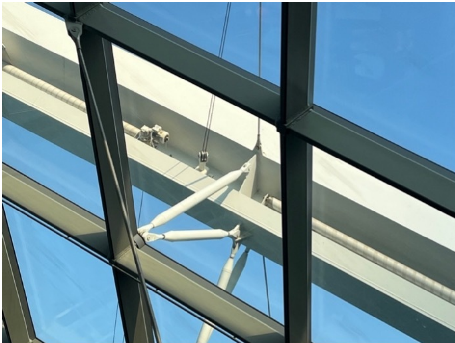
Figure 16: Automated shading panels retract underneath the external structure at the slightest hint of rain or wind. Photo: Nadine Chan.
