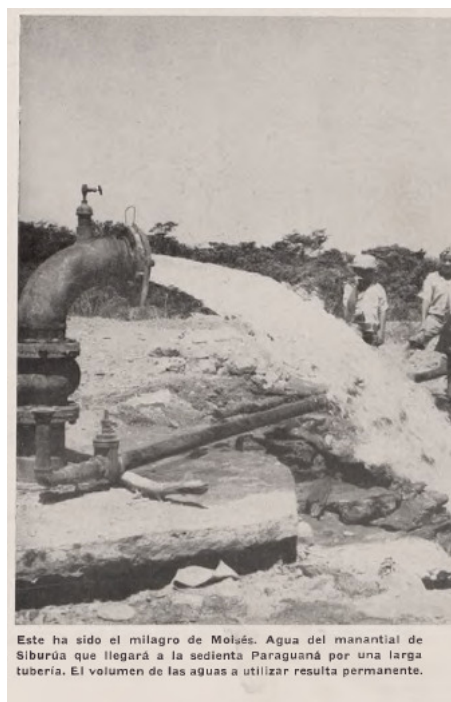
Figure 6: “This has been Moses’s miracle. Water from the Siburua spring arriving at Paraguaná through a long pipeline. The volume of usable water is permanent.”
