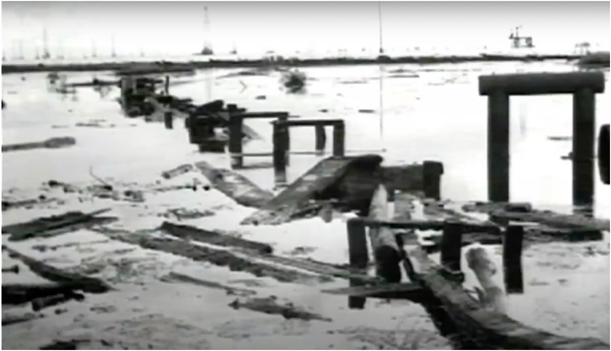
Figure 10: Footage of a dismantled pipeline in Pozo Muerto (1968).
